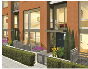
Brix brings 141 new homes, including a limited series of townhouses, to Capitol Hill's Broadway area.
